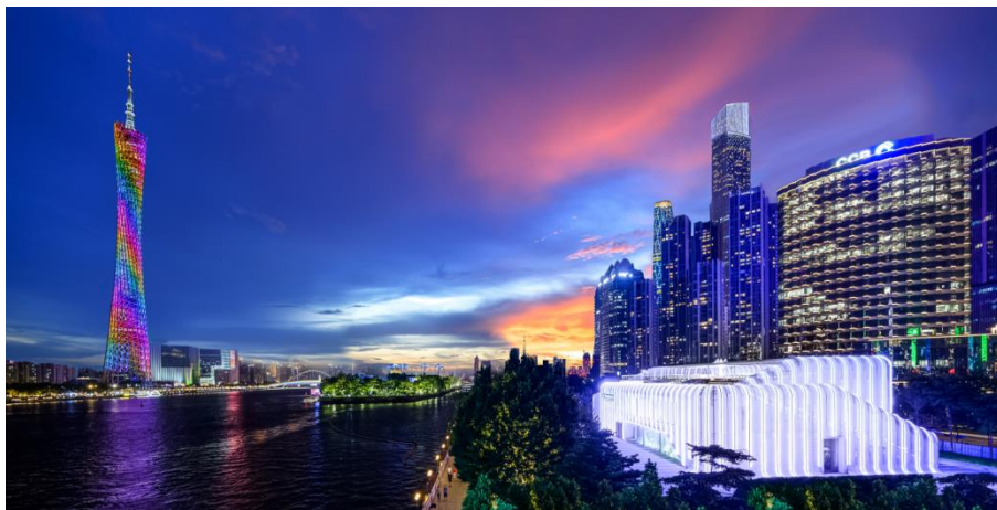
Photo: Guangzhou Transformer Substation Science Popularization Center (110-kilovolt Lieqiao Transformer Substation)
